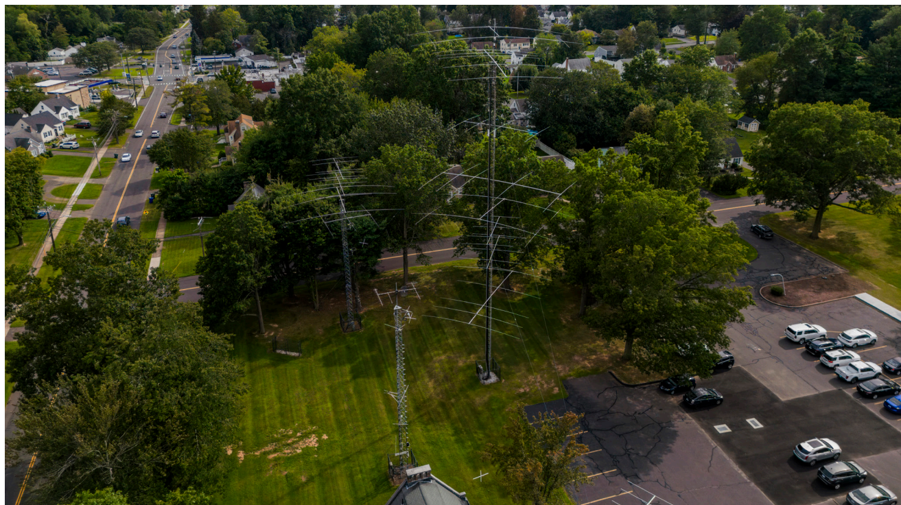
W1AW antennas at ARRL Headquarters.
